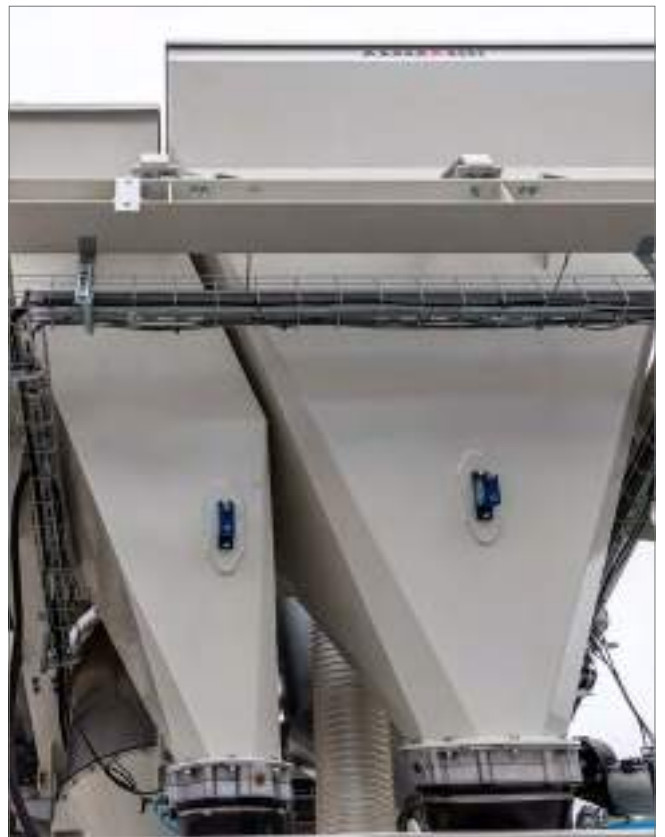
Weighing platform with cement weigher and optional silica weigher.
